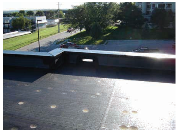
Parapet wall and Scuppers
